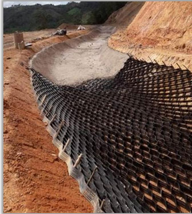
**Figure 18-11: EBP-GV Typical Contact Water Ditch Construction**
