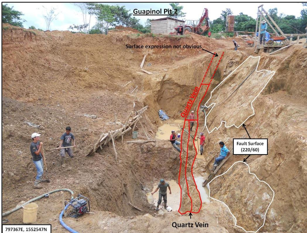
**Figure 9-2: Geological Mapping in Artisanal Mining Pit - – Guapinol Vein, EBP**
